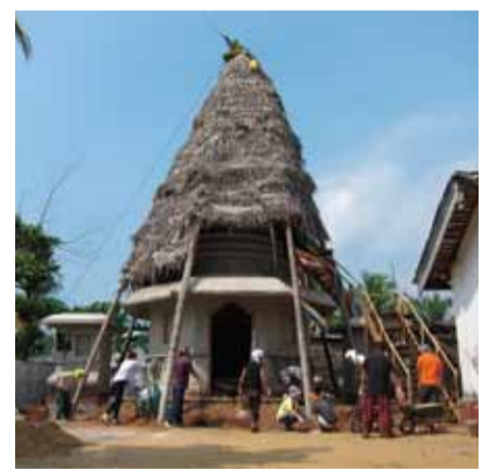
Stupa being constructed
