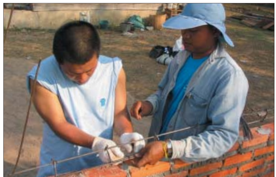
Rev. Tsuo Yokoi (left) reinforces a rod under the supervision of the field supervisor (right)
